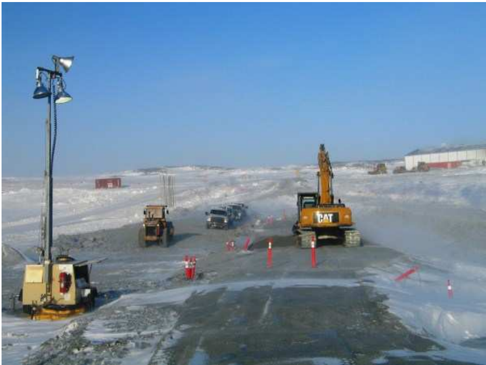
Photo 8: Placing FCM, ~ NNE view.
