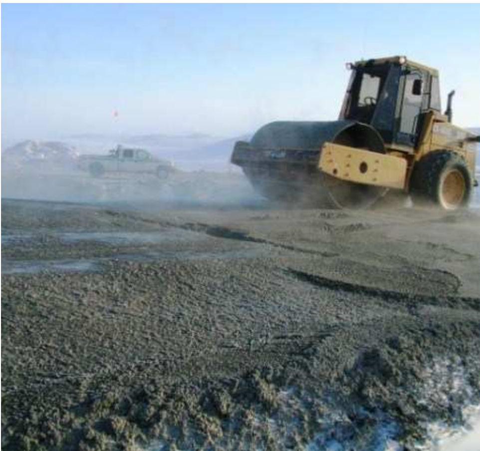
Photo 6: Packing frozen core material, ~ S close-up view.
