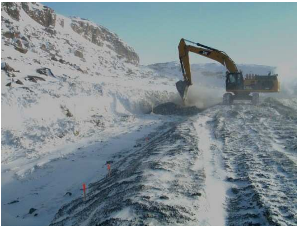
Photo 11: Placing second lift ROQ in key trench Sta 5+30 to 5+85
