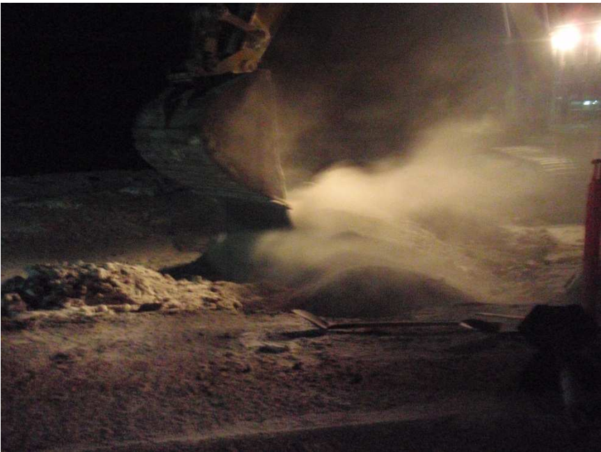
Photo 13: Excavator starting to place ¾" crush around sta 0+85.
