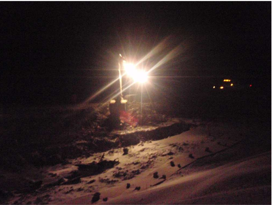
Photo 18: Excavator removing ROQ from upstream inside slope to expose Transition material placed in 2011.
