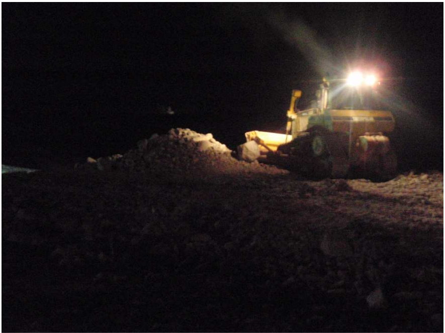
Photo 17: View of D6 spreading ROQ material along downstream
