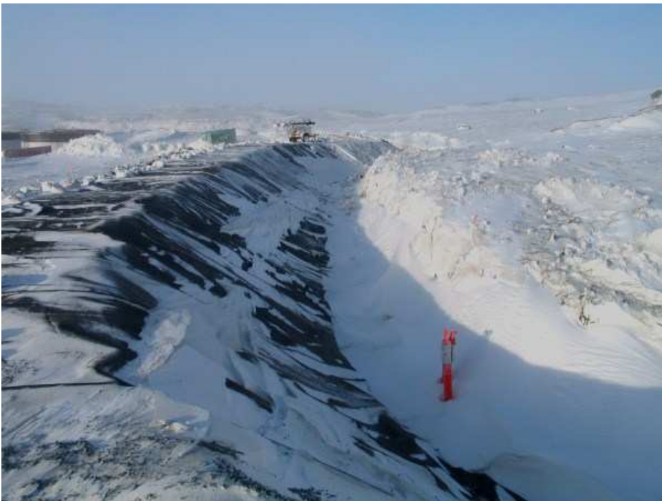
Photo 10: Snow blown in key trench Sta 4+45 facing west.
