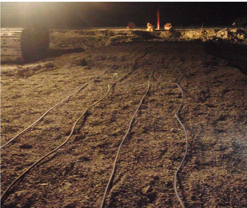
Photo 12: Thermistor cables being laid out around 0+85 in preparation for burring covering cables with additional crush.
