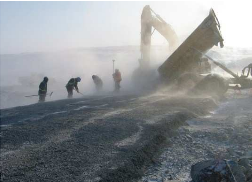
Photo 7: Rakers and surveyor placing FCM
