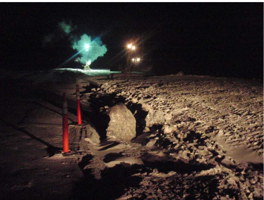
Photo 16: View of a few larger boulders that were bladed to the side as ROQ placement progressed. These were removed from the Transition material footprint on the downstream before additional Transition material placement occurred on nightshift. background shows the location of single bead 27.
